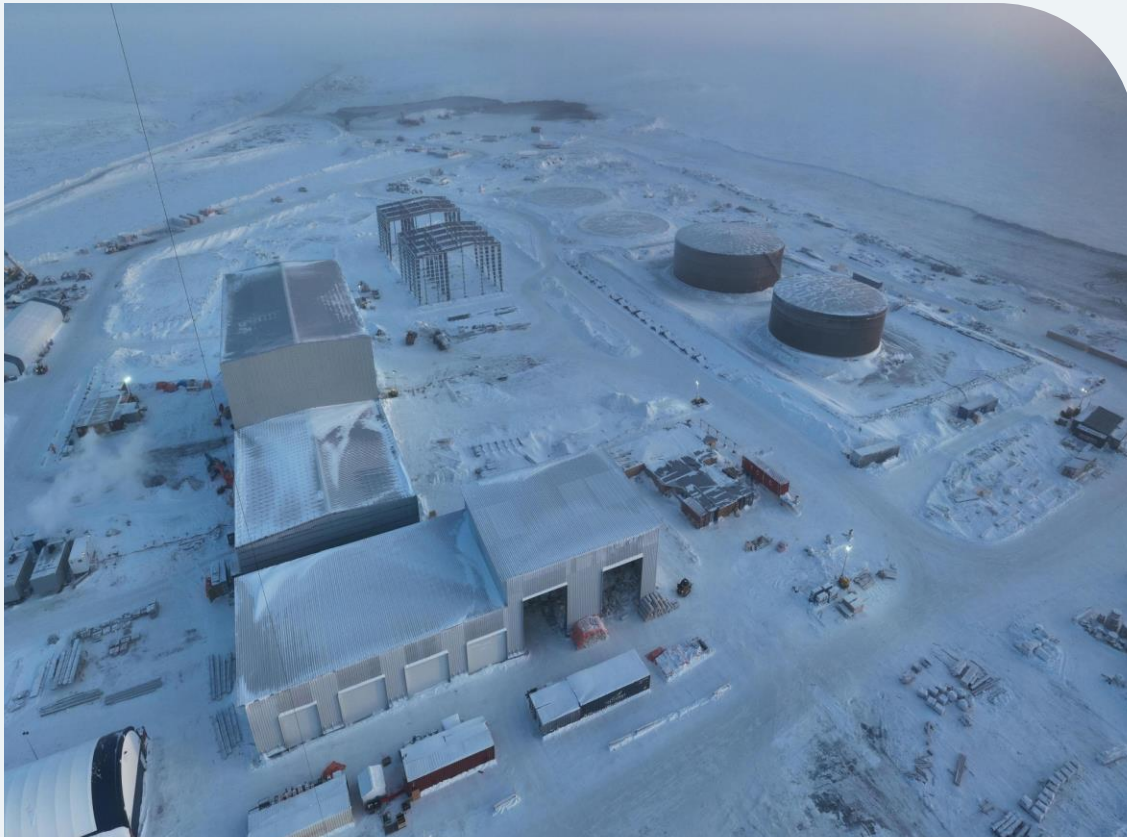
◆ Goose Project Plant Site Area – January 2024
